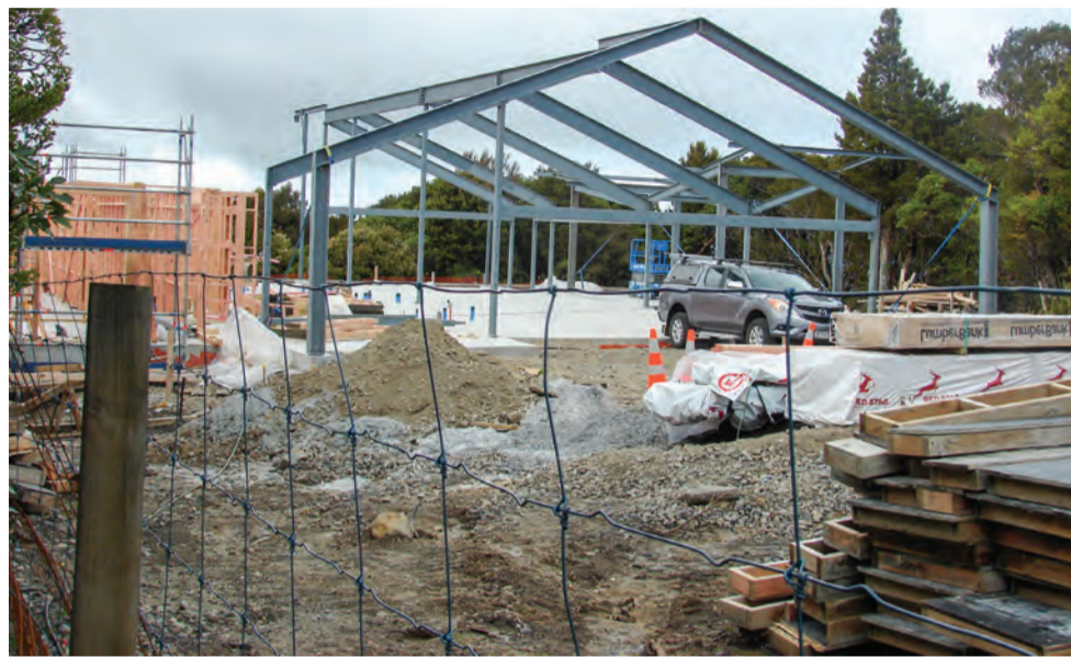
Definite progress is apparent at the Dawson Falls lodge rebuild.
