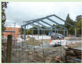
Definite progress at Dawson Falls rebuild. See page 3.
